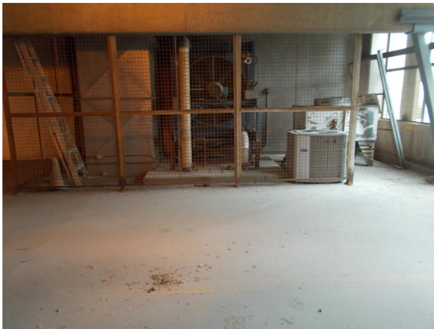
PHOTOGRAPH 22: Showing mechanical equipment located in the Civic Centre Parkade.
