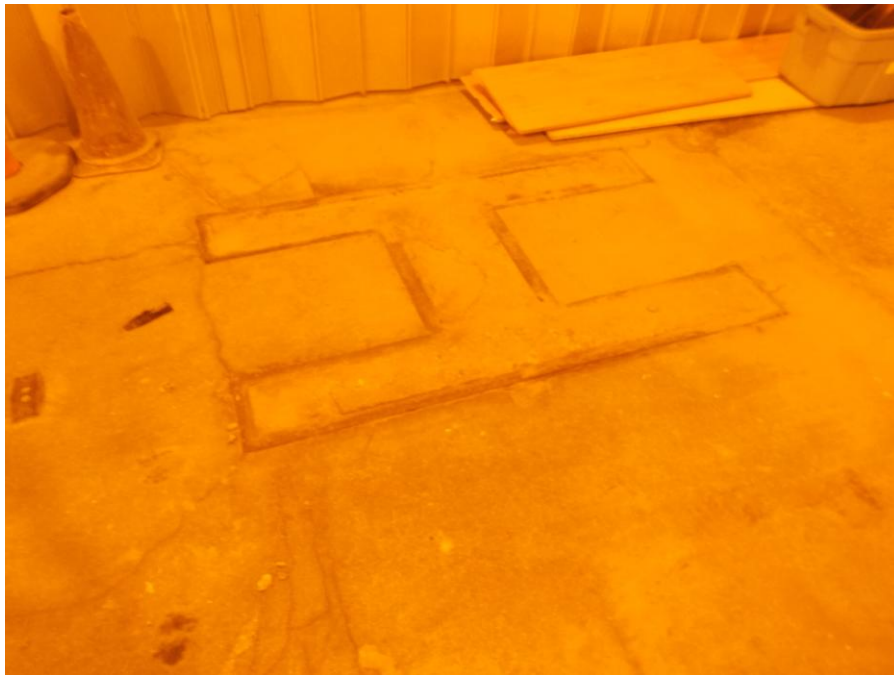
PHOTOGRAPH 17: Showing the inferred former mechanical lift located in the portion of the basement that formally operated as a service area for vehicles.
