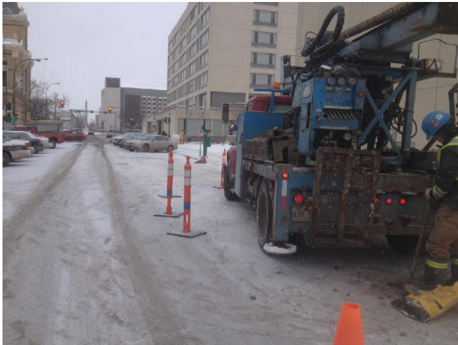
PHOTOGRAPH 5: The drilling of TH13-14 located on James Avenue.
