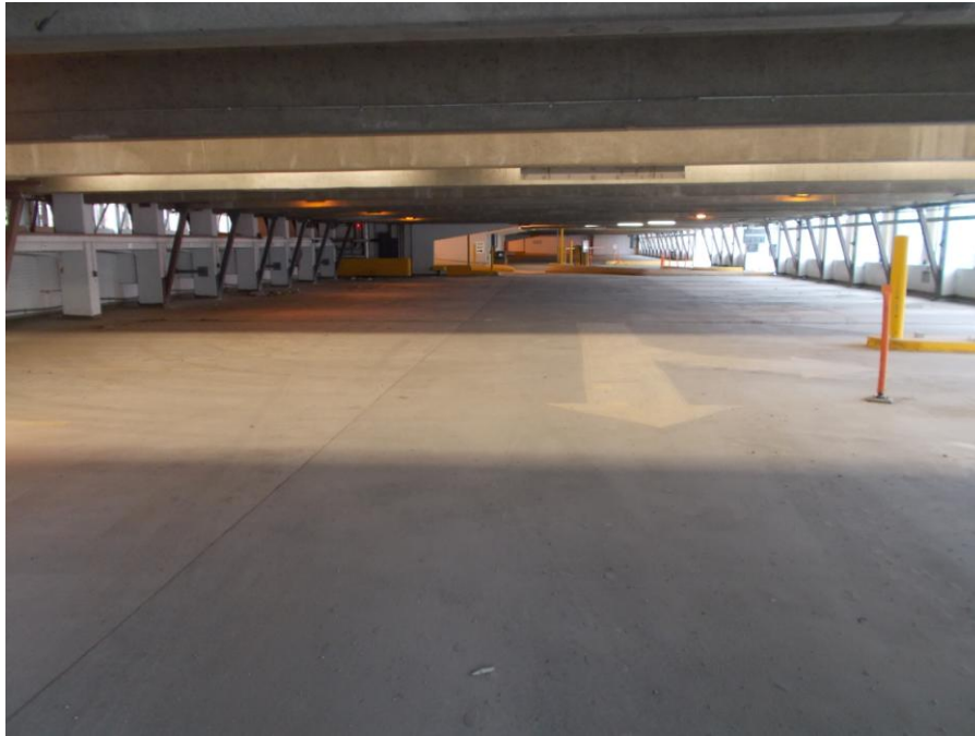
PHOTOGRAPH 21: Showing interior building materials of the Civic Centre Parkade.
