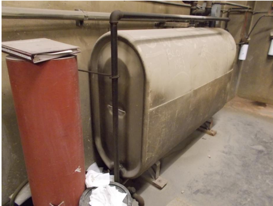
PHOTOGRAPH 19: Showing the day tank located in the basement generator room.
