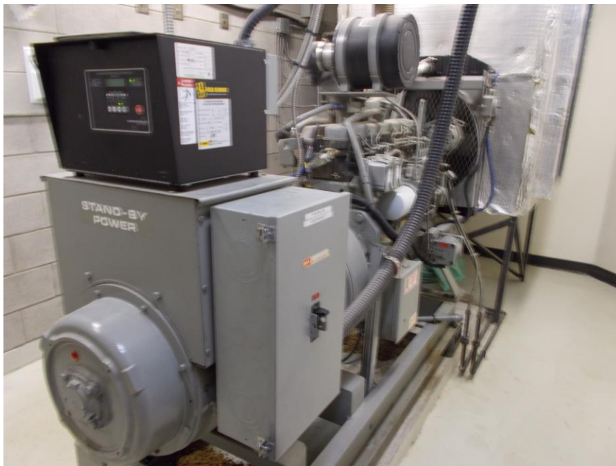
PHOTOGRAPH 12: Showing one of the backup diesel generators located on the 6 th floor.
