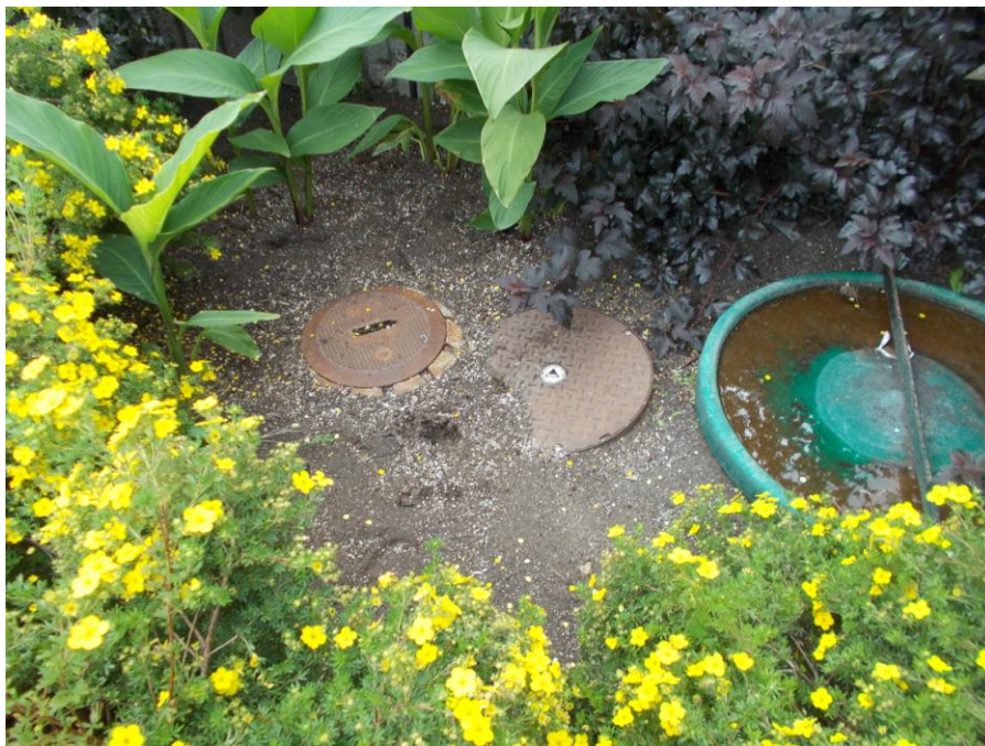
PHOTOGRAPH 20: Showing the fill cap for the 2270 L underground storage tank.
