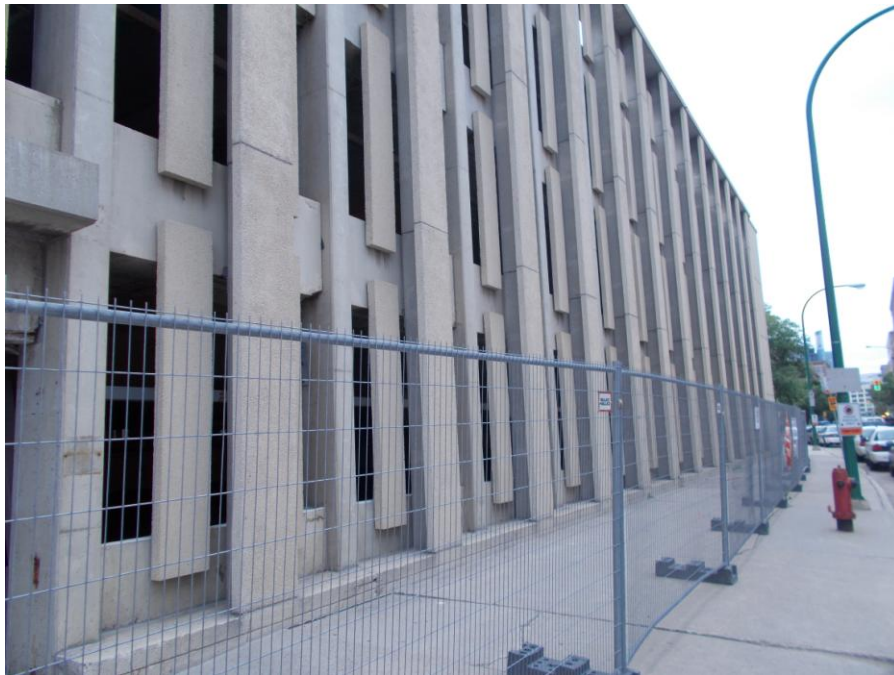
PHOTOGRAPH 3: Looking south /southeast showing the exterior of the Civil Centre Parkade.
