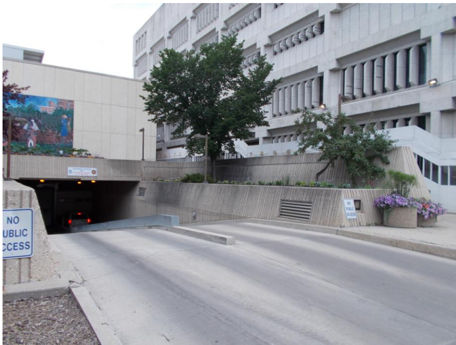
PHOTOGRAPH 4: Looking northeast across the Site from the entrance to the basement level of the Site buildings.
