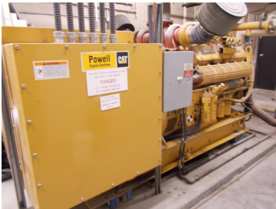
PHOTOGRAPH 18: Showing the backup generator located in the shared basement of the Site buildings.
