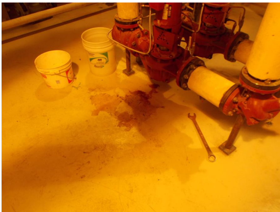
PHOTOGRAPH 14: Showing an example of the surface staining that was observed on the 6 th floor.
