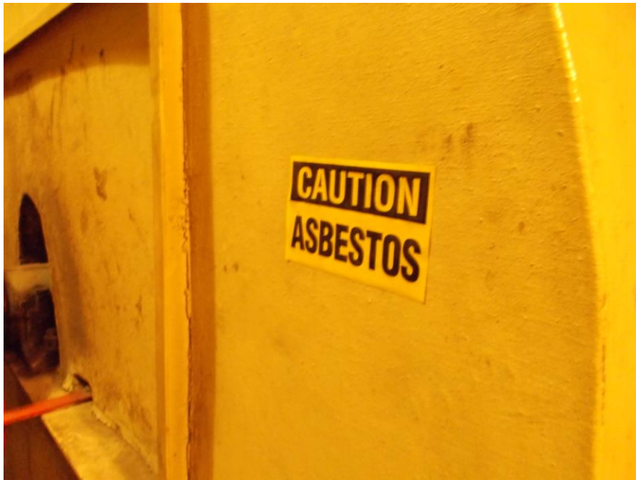
PHOTOGRAPH 11: Showing an example of asbestos labelling within the Site buildings.
