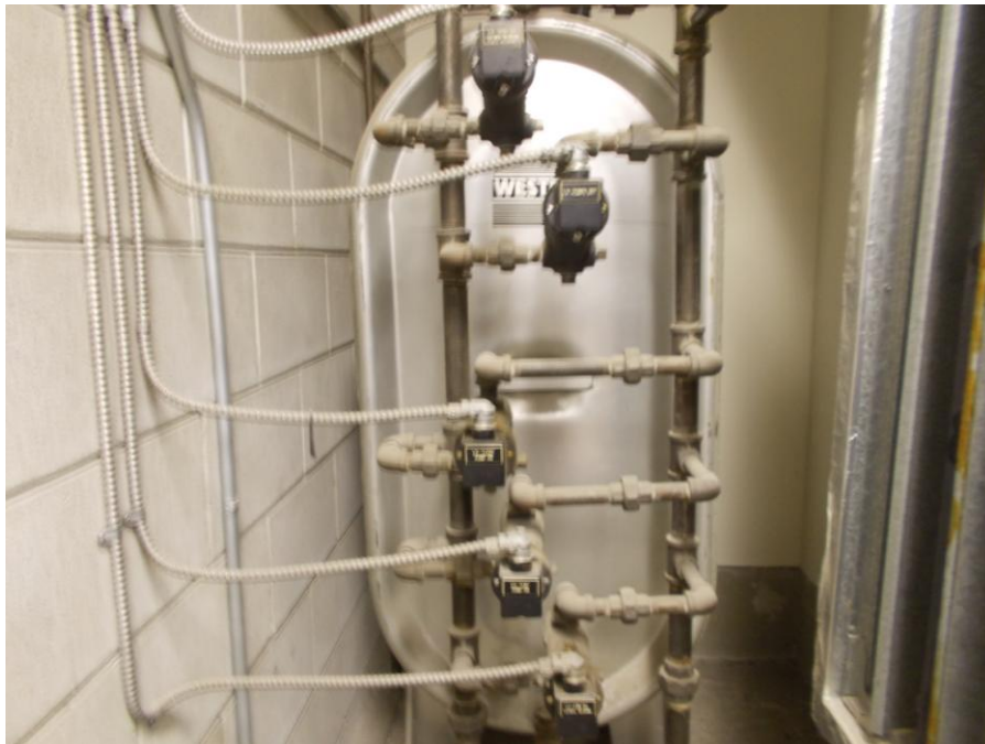
PHOTOGRAPH 13: Showing the diesel day tank located on the 6 th floor in generator room 1.
