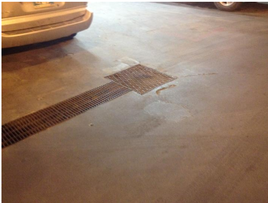
PHOTOGRAPH 2: The floor drain located within the basement of the parkade. TH13-04 was advanced near this location.
