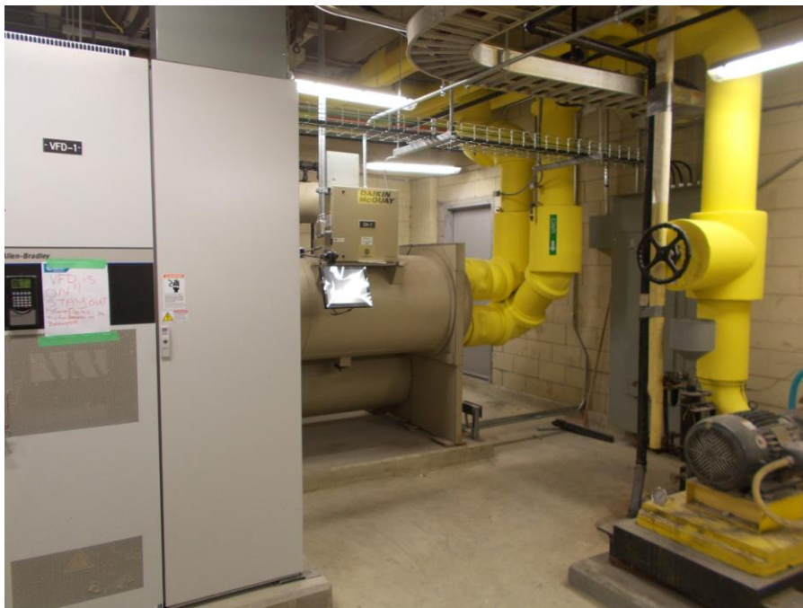
PHOTOGRAPH 10: Showing typical building materials observed on within the 6 th floor mechanical rooms.
