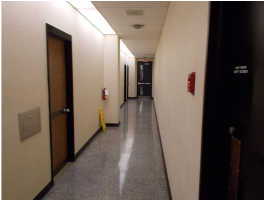
PHOTOGRAPH 7: Showing the typical interior building materials of the Public Safety Building.
