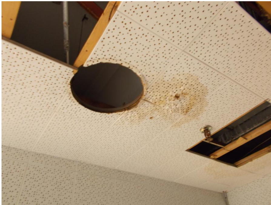
PHOTOGRAPH 15: Showing water damage observed in the basement located below the Civic Centre Parkade.
