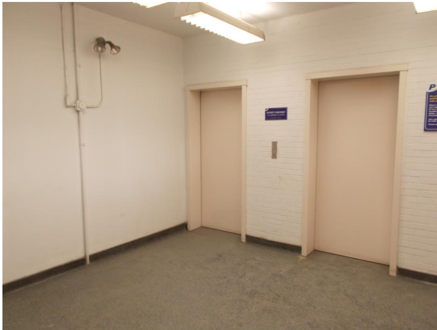
PHOTOGRAPH 23: Showing the interior building materials of the stairwells / elevator access areas of the Civic Centre Parkade.
