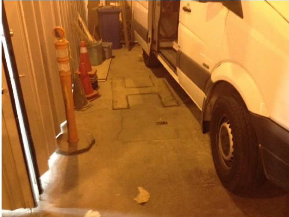
PHOTOGRAPH 1: The inferred former hydraulic joist. TH13-01 was advanced near this location.
